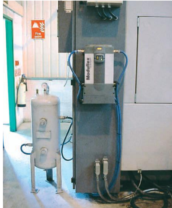
Moduflex Dry Air System installed to supply control air for a CNC machining centre
